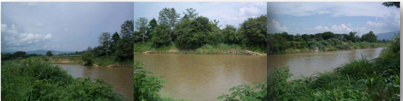
River Front View East - South - West
